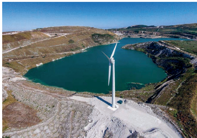
This wind turbine installed by Imerys in its Blackpool quarry (Cornwall, UK), supplies 180,000 kWh a month of cost-efficient low-carbon energy © Imerys
