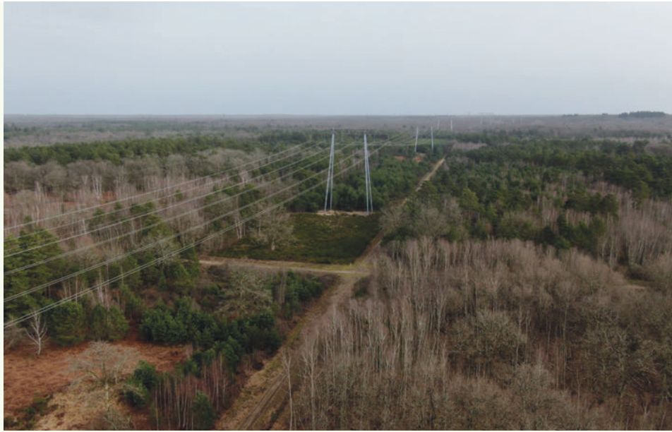
Power line maintenance site carried out in 2021 in the Loiret
