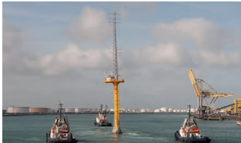
Measuring mast at the entrance to Le Havre port as part of the Fécamp wind farm project. ©EOHF - Laurent Critot
