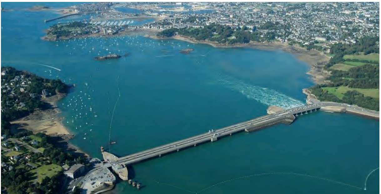
Rance tidal power station. © EDF
