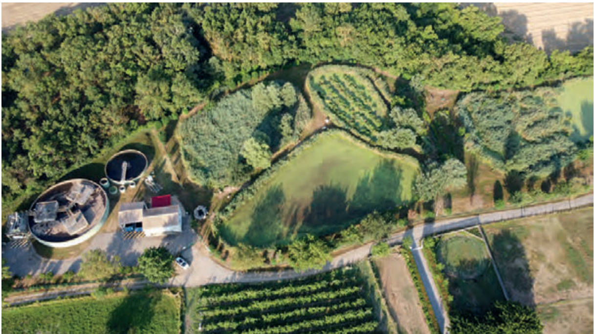
The Dragonfly Zone (Zone Libellule) for «Biological Freedom and Tackling Emerging Pollutants» connected to a wastewater treatment plant - ZHART project (Wetlands) - SUEZ
